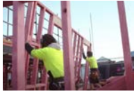
Pre-fabricating wall frames before standing them up
