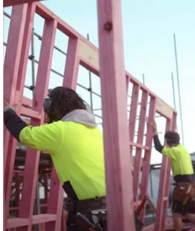
Pre-fabricating wall frames before standing them up
